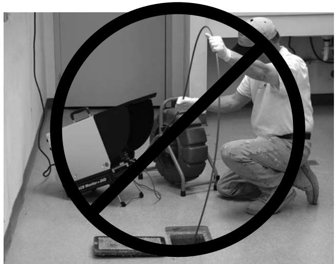
Figure 27 – Improper Cable Push
