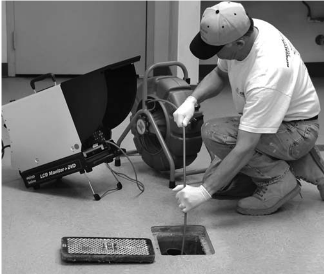
Figure 28 – Proper Cable Push
